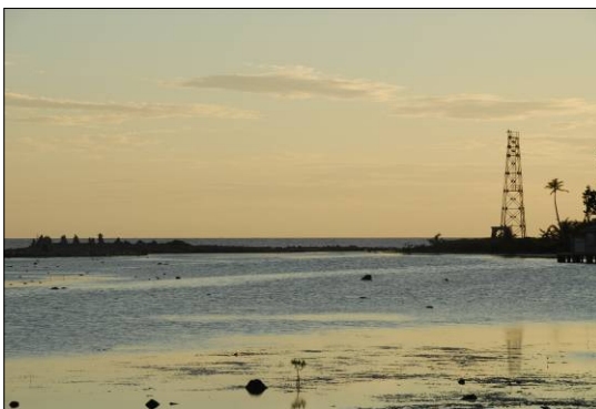
Figure 28: Lighthouse on Southwest II Caye
